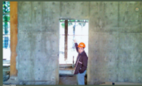
Seismic Option 1 - Shear Wall Construction
