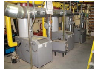
CONDENSING HOT WATER BOILERS
