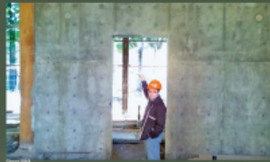
Seismic Option 1 - Shear Wall Construction
