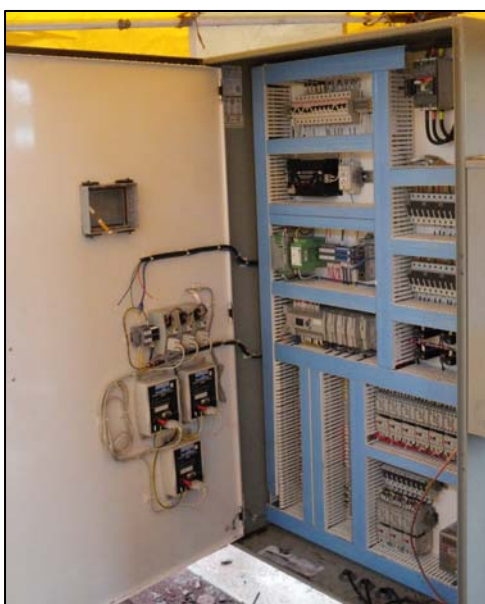
Control System Electrical Panel
