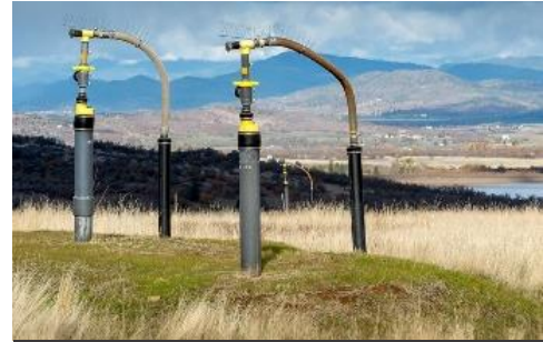
A landfill gas well at Dry Creek Landfill in Eagle Point, Oregon.
