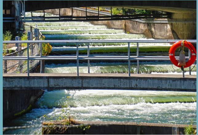
Fish ladder at the Bonneville Lock and Dam. Photo: U.S. Army Corps of Engineers, Portland Corps.
