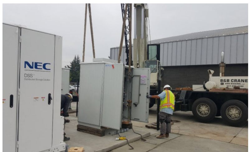
EWEB contractor installs back-up battery power system.
