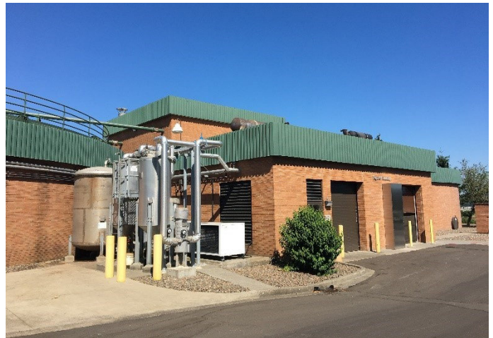
Gresham Wastewater Treatment Plant
